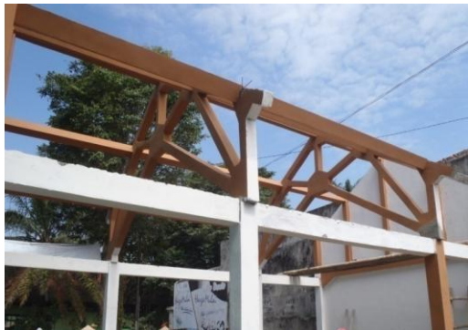
Figure 3 Precast bamboo reinforced concrete roof frame
