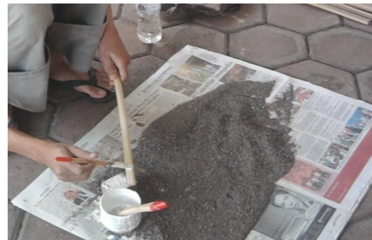
Figure 1 Painting and smear bamboo reinforcement
